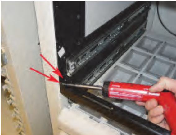
Figure 5-48. Installing the bottom crossbar
