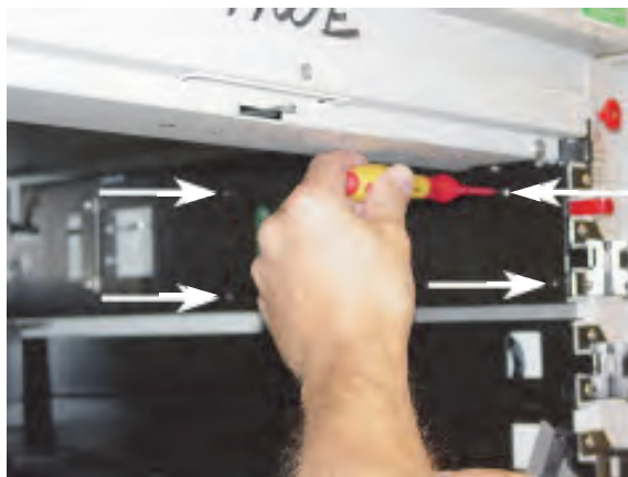
Figure 5-83. Securing the carrier controller cover
