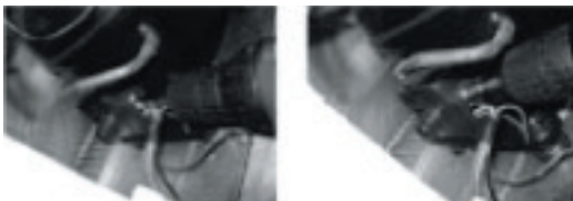
(2) Remove two screws on comp base
