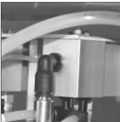
Drive gas connection for individual pipeline manifold
