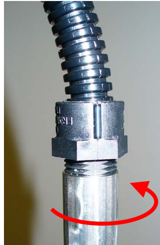
Pic. 48a Screwing of the clip into the conduit
